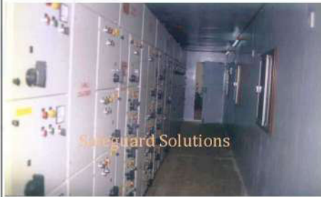
Control Room Bunk House
