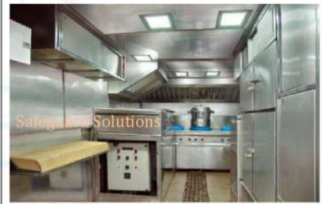
VFJ Kitchen Bunk House Interior
